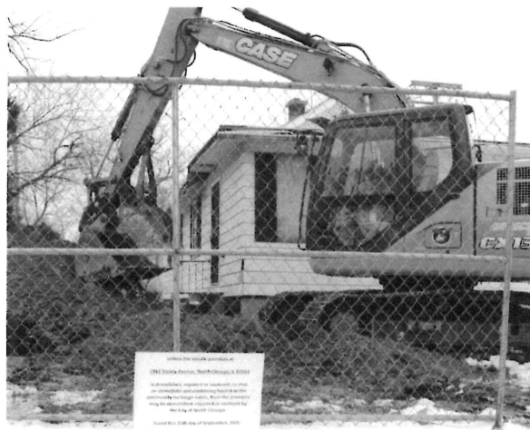
The blighted house at 1912 Dickey Avenue was demolished on January 6, 2021.
